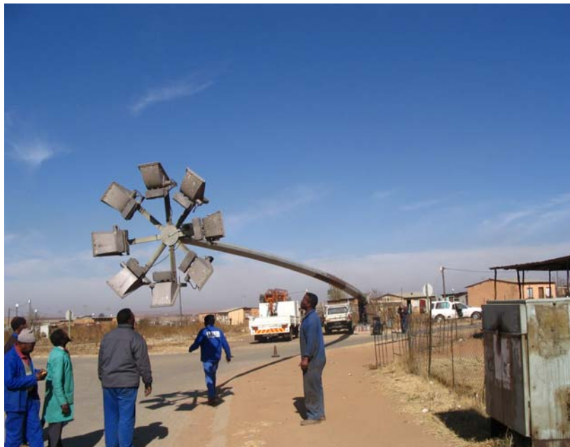
Installing 11High Mast Lights Ext 23
