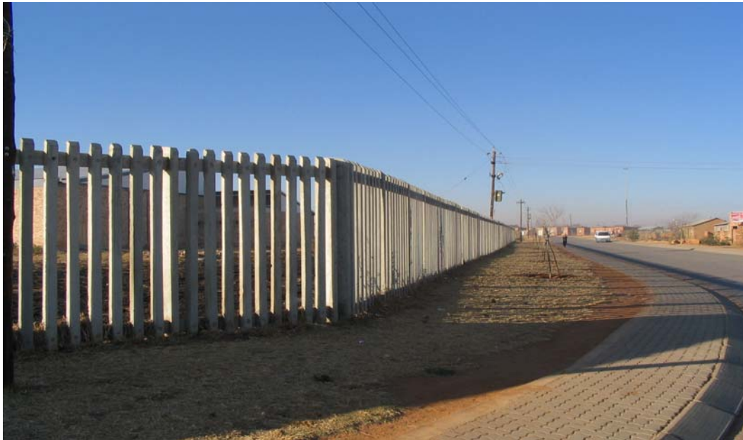
Completed Fencing Ratanda Ext 7
