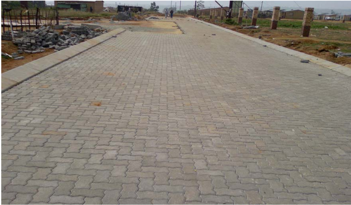
Laying of bedding, Kerbing and Paving @ Blackwood Avenue.
