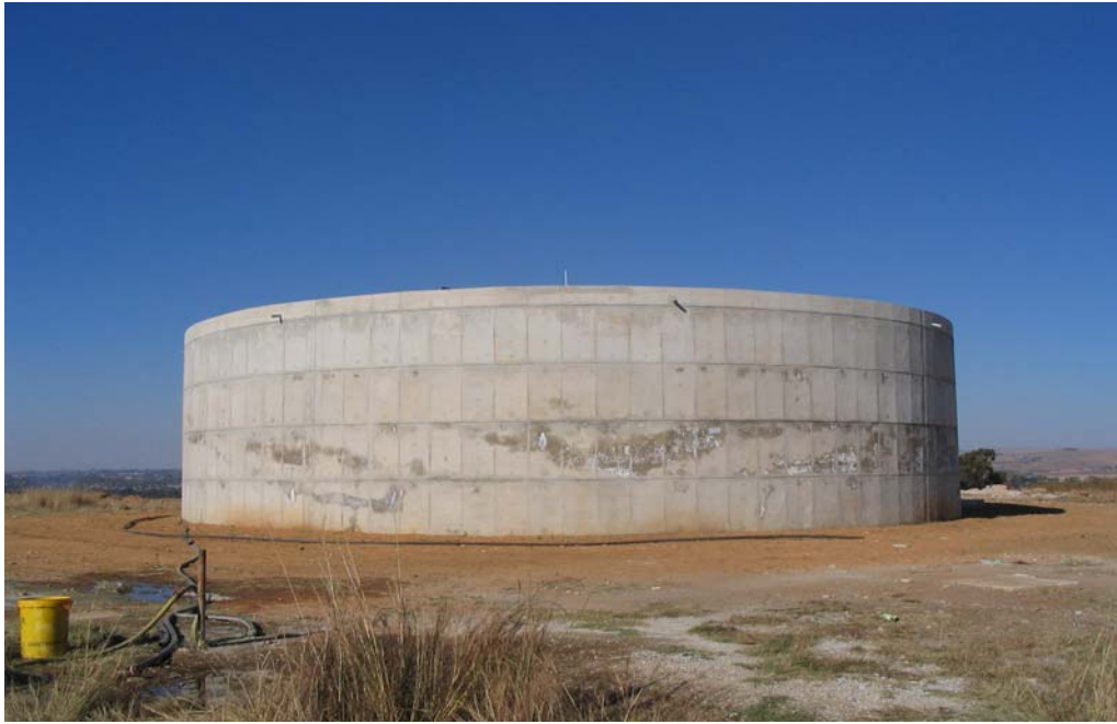
Completed a New 1.5 Megalitre Reservoir in Jameson Park
