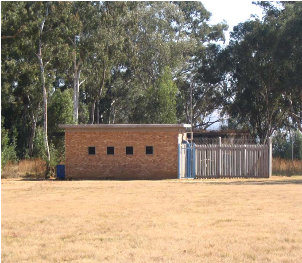
Install New Water Bulk Supply Pipeline and Pump station Ext 23
