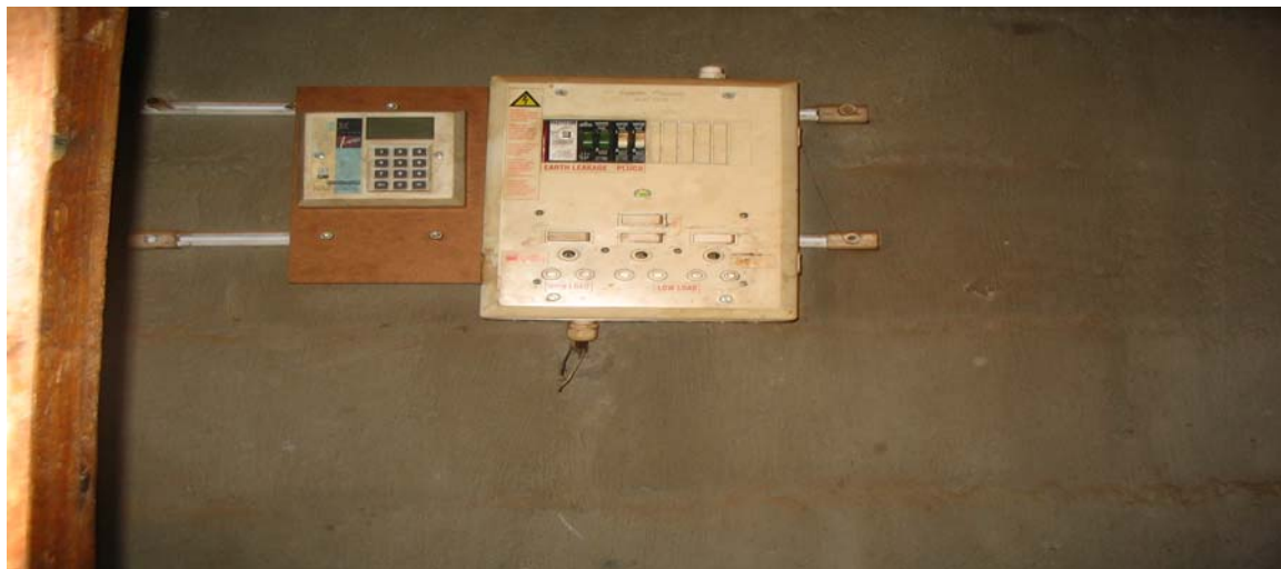
Electrification of 750 stands of Tokolohong and Ext 23
