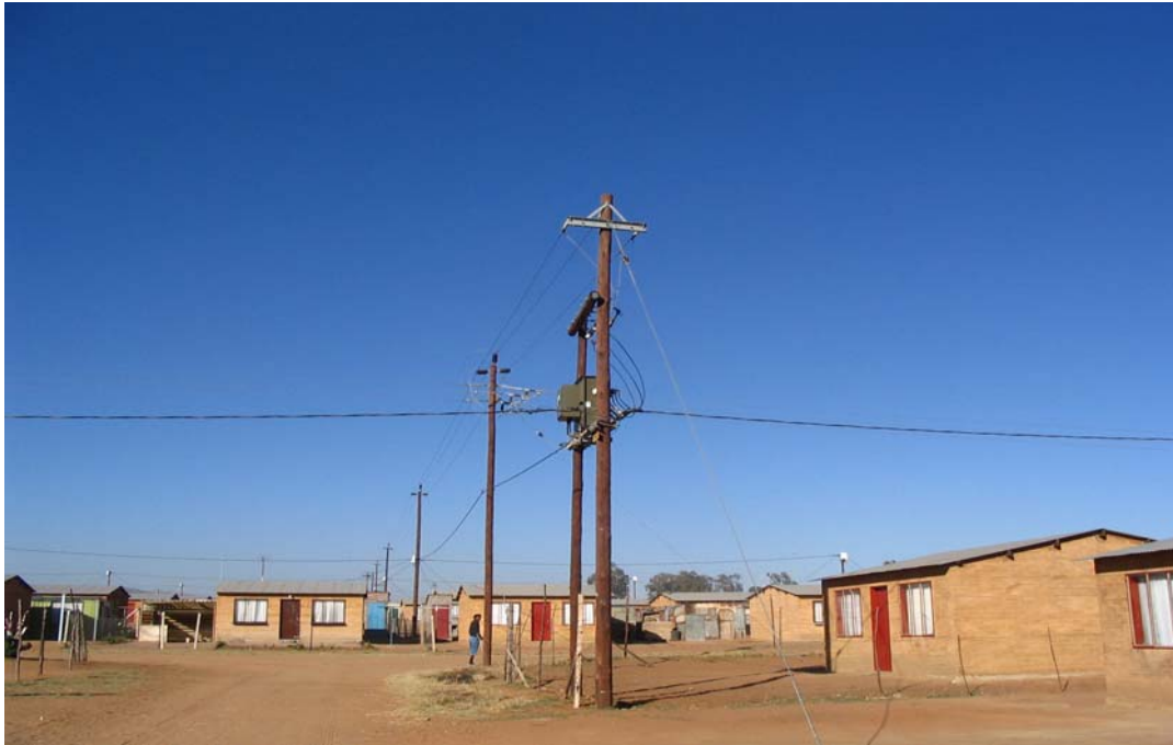
Electrification of 750 stands of Tokolohong
