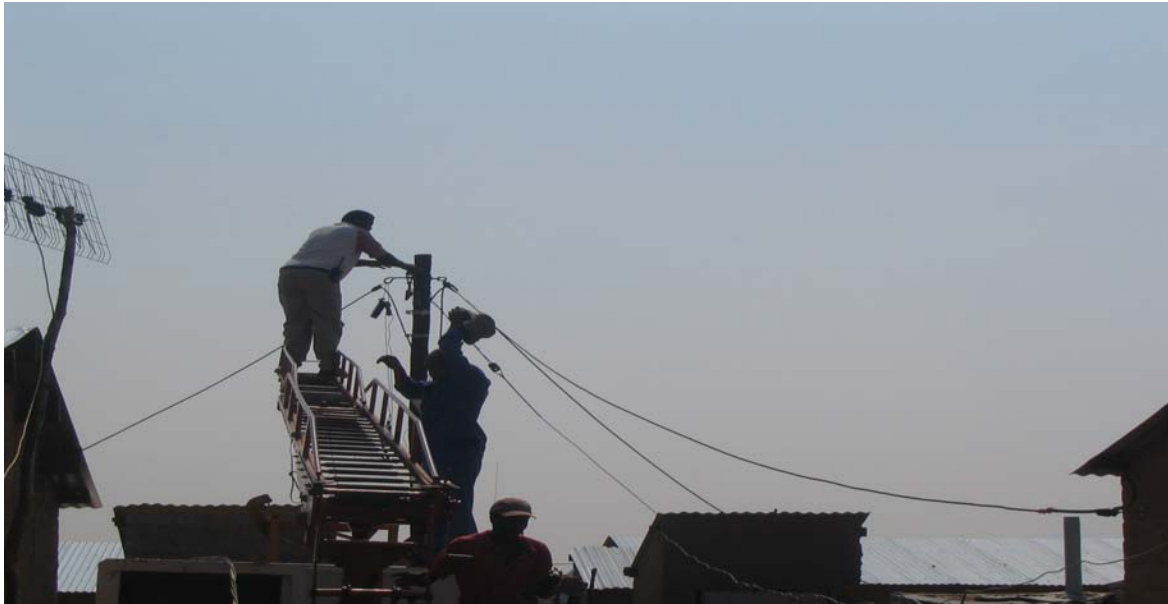
Electrification of 750 stands of Tokolohong and Ext 23
